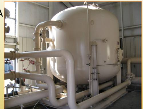
A 'Model 12' vessel filled with 740 ft<sup>3</sup> of GAC for DBCP removal. Almond shell GAC filter columns were installed at the inflow to this vessel.
