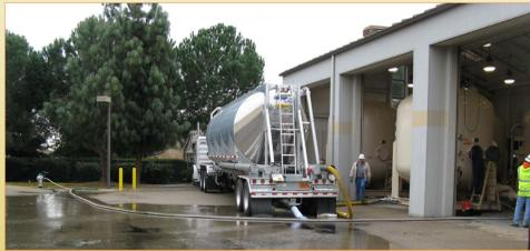
Changing spent carbon from GAC vessels requires good coordination of labor, new materials and water system requirements.
