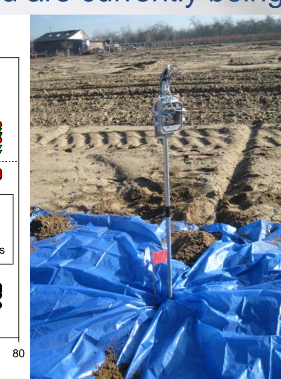
Figure 4: Hobo dataloggers (right) were used to record soil temperature at 12 and 24-inch depths in steam-disinfested future tree sites. The target temperature of 158F was usually exceeded for at least 30 minutes after the steam injection (left)
