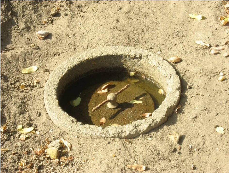
Figure 7. Orchard Irrigation Valves Along South Side of Orchard
