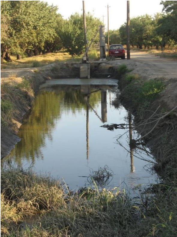
Figure 5. Sediment Basin in Northeast corner of Orchard
