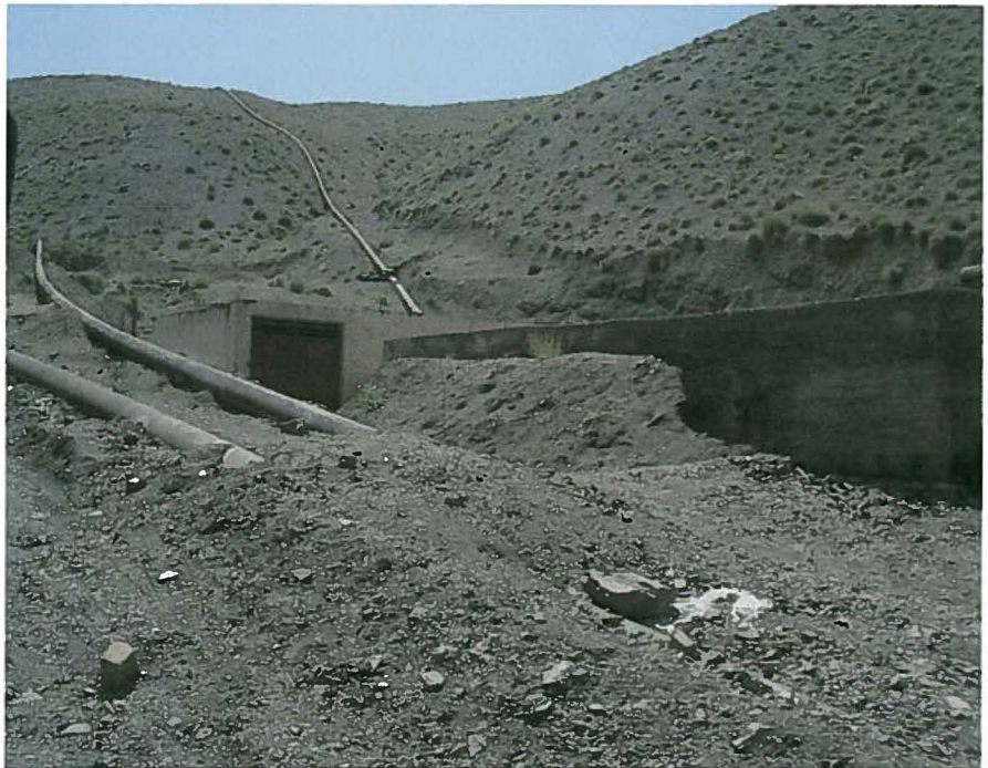
Figure 26. One of several pumping stations required to deliver irrigation water to the high elevation almond orchards.
