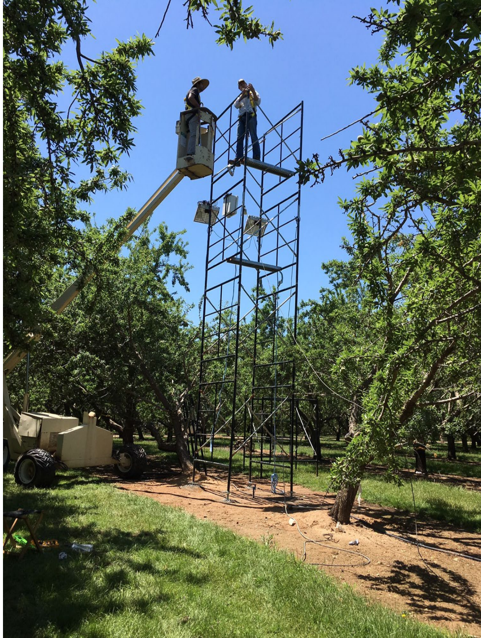
Figure 6: New Flux tower installation at Nickels Ranch, where collaborator Tom Buckley is conducting sap flow measurements on trees in an experimental orchard.
